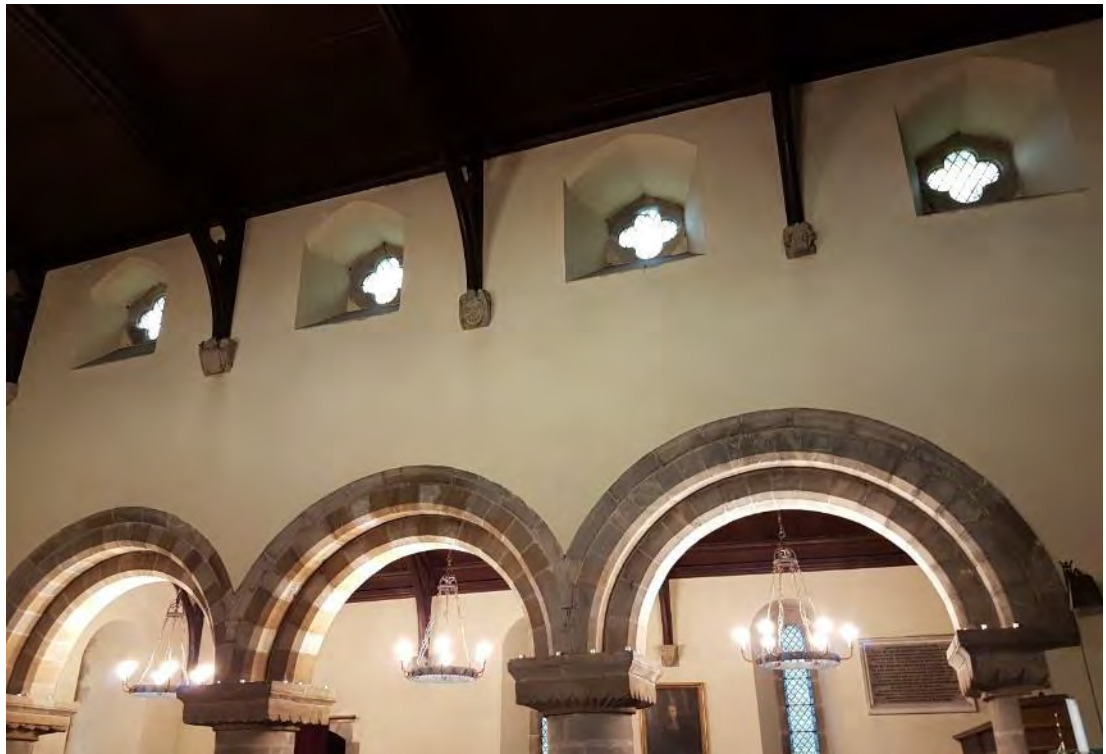
Figure 40: The C15 corbels along the north wall of the clerestory, decorated with family crests and human heads. The corbels are interspersed between clerestory windows of quatrefoil tracery set inside a chamfered segmental pointed arched surround and chamfered sill (Source: Author 2019).
