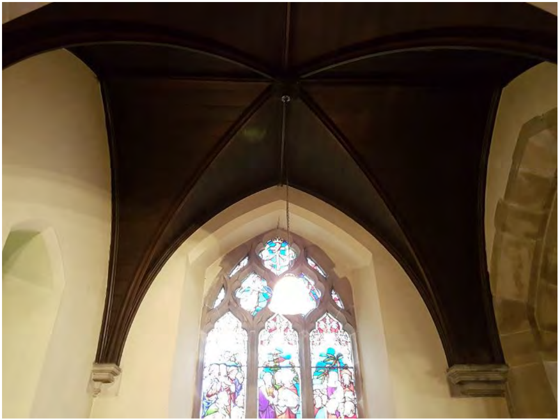
Figure 89: The quadripartite timber ceiling of the vestry resting on limestone corbels (Source: Author 2019).
