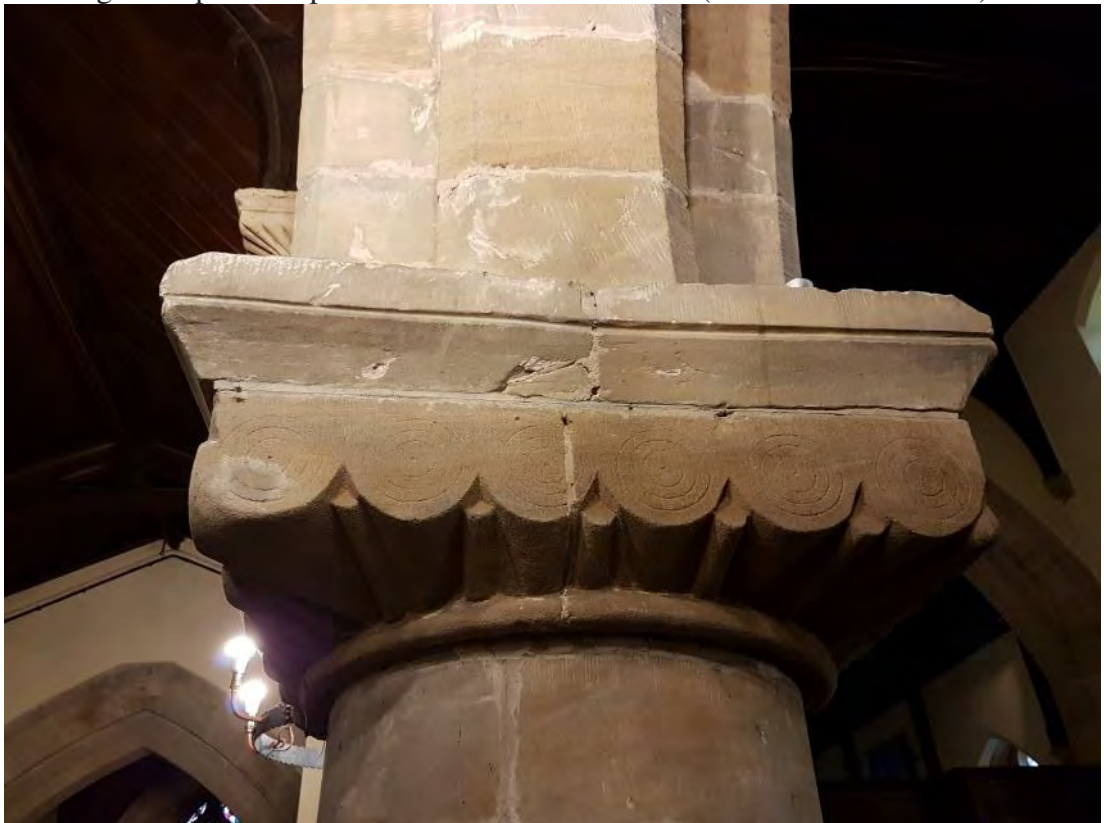
Figure 22: The capital of the eastern pillar of the central bay of the northern arcade, showing scalloped trumpets with incised medallions ready for decoration (Source: Author 2019).
