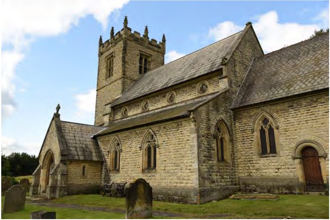
Figure 67: The eastern elevation of the porch (Source: Author 2019).
