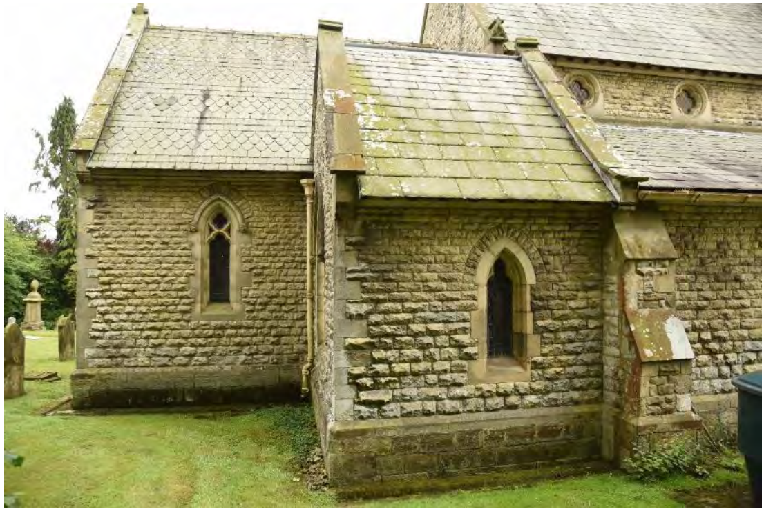
Figure 93: The northern elevation of the chancel and the chancel bay of the north aisle, showing the window on the northern elevation of the chancel to be a cusped one-light Geometric Decorated pointed arch window with quatrefoil tracery and rounded hood-moulds with head-stops (Source: Author 2019).
