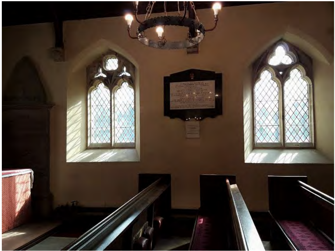
Figure 60: The eastern end of the south aisle, showing from the left: the C17 altar; a C19 memorial tablet; an 1862-3 Victorian Middle Gothic pointed arch window of the western bay; a C19 memorial tablet with a Victorian lamp retrofitted with electricity; an 1862-3 Victorian Middle Gothic pointed arch window of the middle bay; and, C19 pews below (Source: Author 2019).
