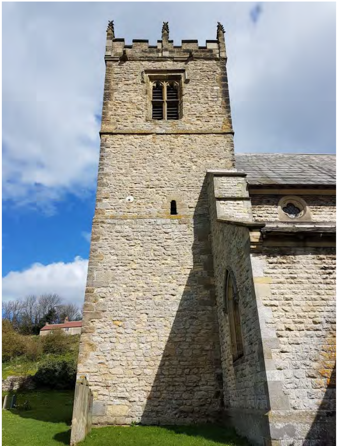
Figure 111: The southern elevation of the three-stage square tower, constructed from coursed rough limestone rubble with dressed calcareous sandstone quoining, with the Norman window in the second stage (Source: Author 2019).
