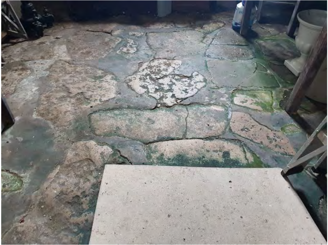
Figure 127: The stone and cementitious mortar flooring of the first stage of the tower (Source: Author 2019).
