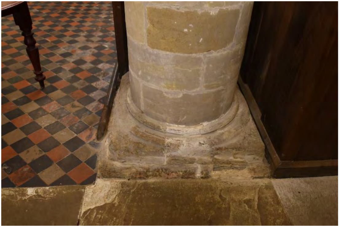
Figure 25: The base of a typical column along the northern arcade, comprising a circular torus on top of a scotia, circular chamfered torus and a square base, on top of a square plinth (Source: Author 2019).
