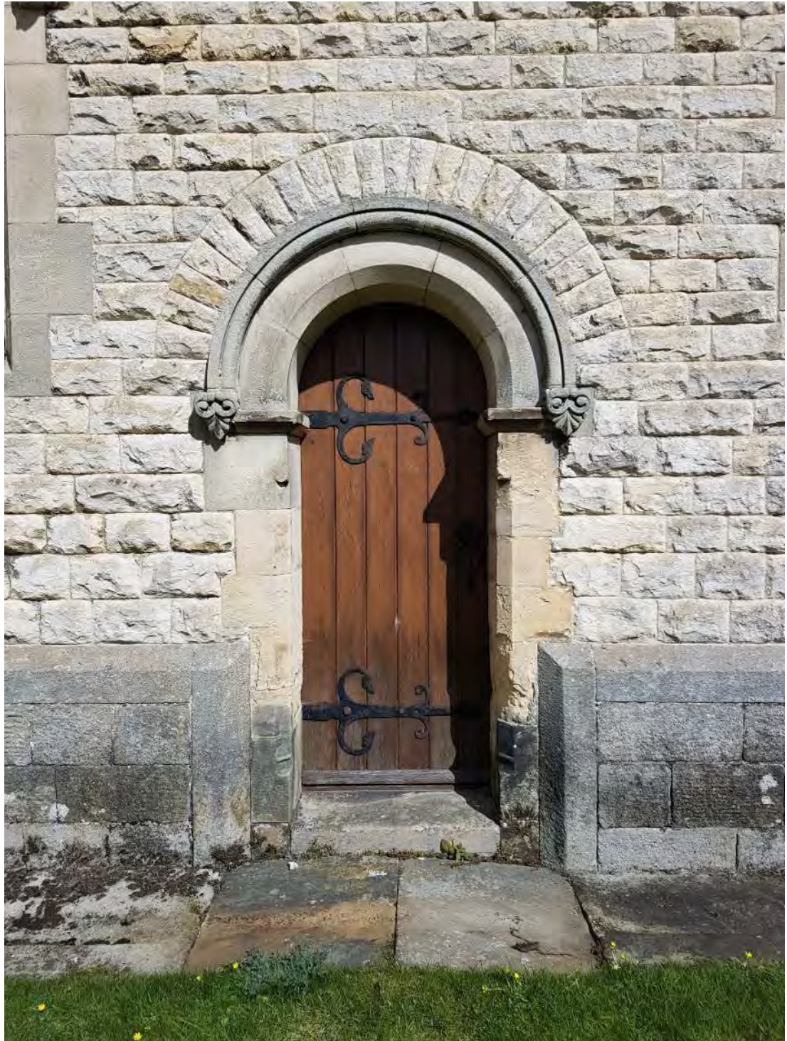
Figure 94: The Victorian interpretation of a Norman narrow rounded-arched door with chamfered quoining and a rounded hood-mould with floriolate label-stops in the central bay of the southern elevation of the chancel (Source: Author 2019).
