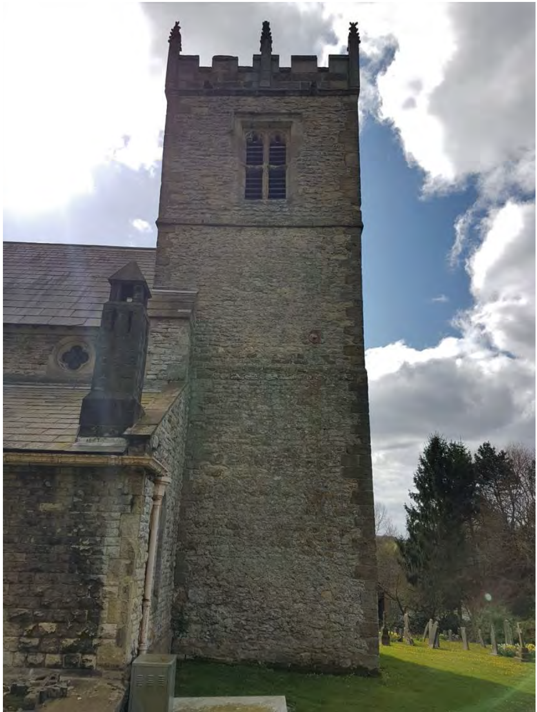
Figure 109: The northern elevation of the three-stage square tower, constructed from coursed rough limestone rubble with dressed calcareous sandstone quoining, with the first two Norman stages and the fifteenth-century Perpendicular belfry (Source: Author 2019).
