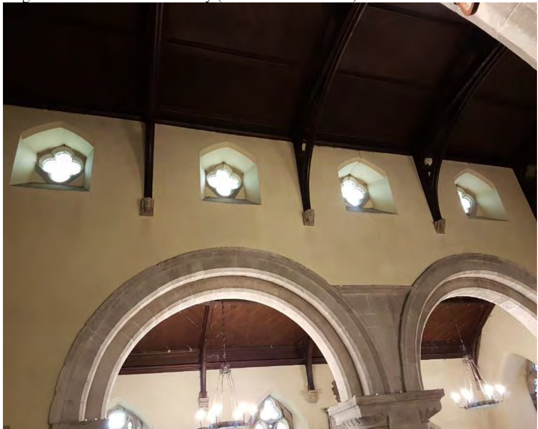
Figure 163: The extant clerestory windows in the south aisle, showing the reused, deeply sloping sills of the fifteenth-century clerestory in the same location as the previous windows, with the corbels at a lower height than their C15 location (Source: Author 2019).
