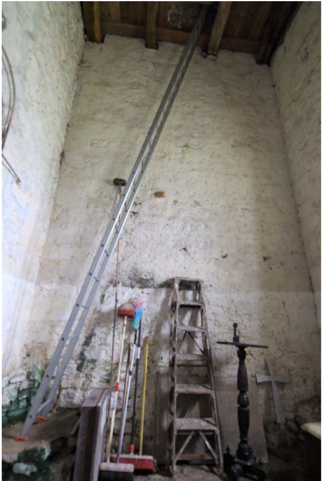
Figure 119: The interior of the first stage of the tower, looking south at the southern wall, showing the painted coursed rubble stone masonry (Source: Author 2019).
