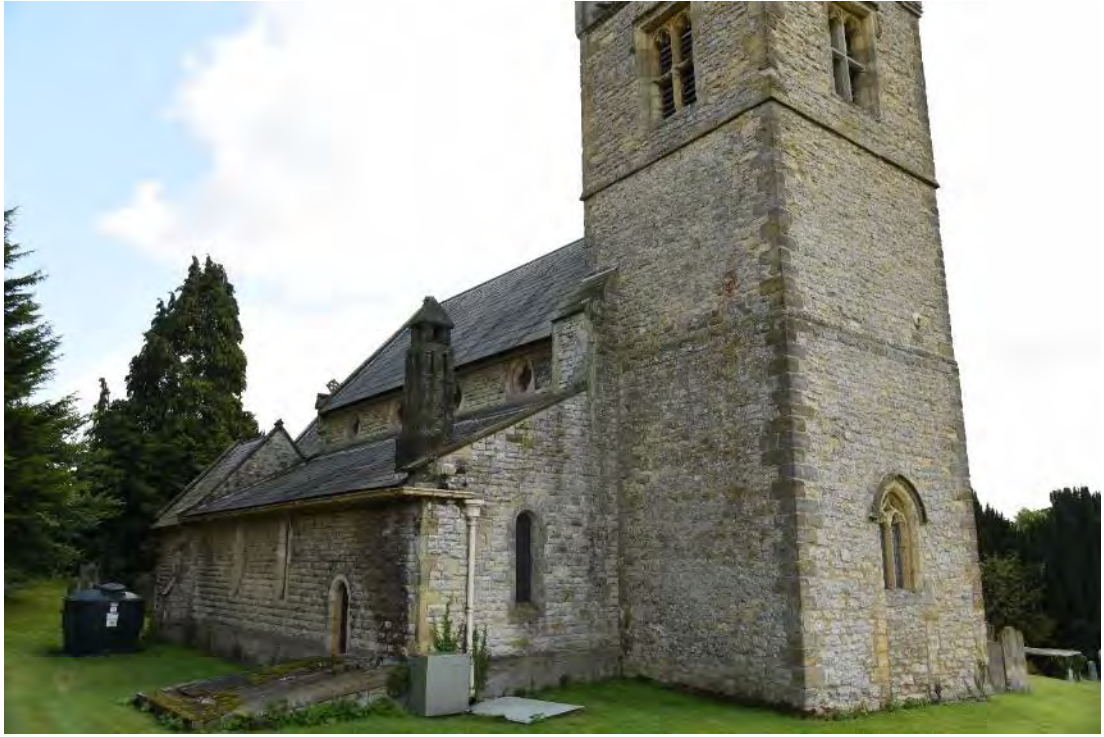
Figure 8: The northern and western elevation of Stonegrave Minster from the north-west (Source: Author 2019).
