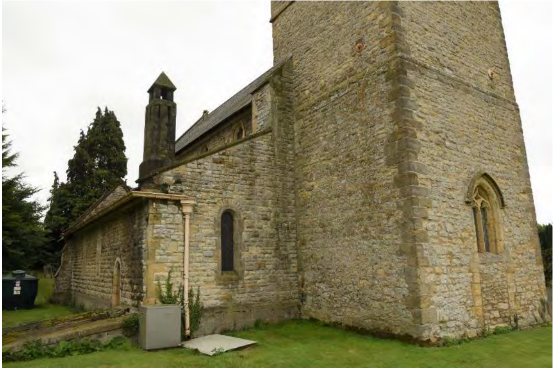
Figure 73: The western elevation of the north aisle abutting the western tower, showing the one-light lancet window (Source: Author 2019).
