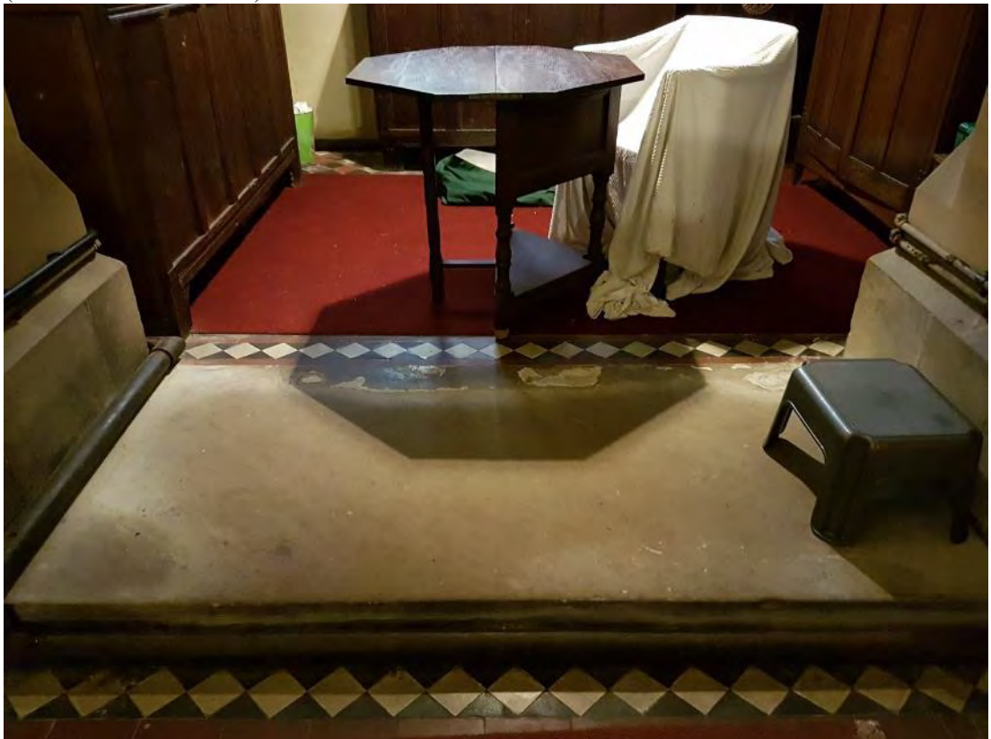
Figure 90: The floor of the vestry/chancel bay of the north aisle, showing the stone slab threshold within the arch with flanking geometric tiles and carpet (Source: Author 2019).
