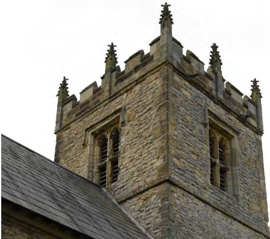
Figure 116: The northern and eastern elevations of the third stage of the tower, showing fifteenth-century Perpendicular louvred windows and an embattled parapet topped with Victorian pinnacles based on fifteenth-century precursors (Source: Author 2019).
