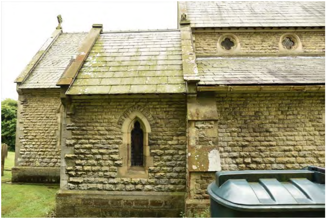
Figure 75: The northern elevation of the vestry, or chancel bay of the north aisle, showing the one-light Victorian window and the graduated buttress between the nave and chancel bays (Source: Author 2019).
