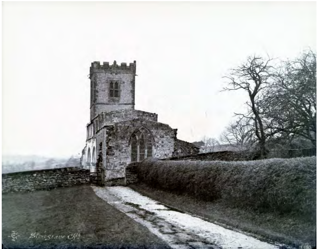
Figure 136: Photograph of the eastern elevation during the demolition in 1862-3, showing the C18/early C19 intersecting y-tracery of the eastern window, the C15 roof structure of the chancel and nave, looking west (Source: NSM RPS 18950).
