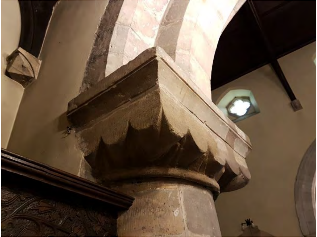
Figure 21: The capital of the eastern pillar of the eastern bay of the northern arcade, showing scalloped trumpets with no floral medallions (Source: Author 2019).
