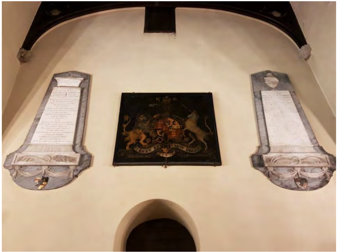
Figure 38: The western wall of the nave and eastern side of the eastern wall of the tower, showing the top of the arched doorway, the two early C19 mural tablets flanking the coat of arms, the reused C15 corbels and the western side of the upper door in the tower (Source: Author 2019).
