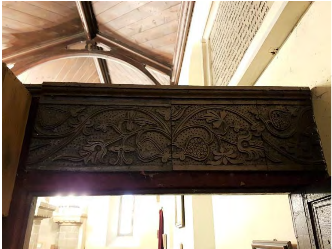
Figure 183: The back of the reused seventeenth-century screen running between the eastern nave bay and chancel bay of the north aisle, taken from the vestry, showing the reused floriated frieze above the door (Source: Author 2019).
