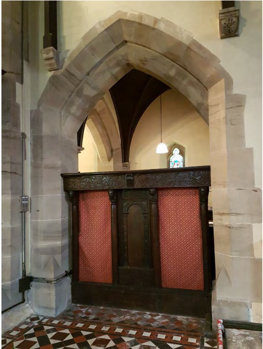
Figure 78: The Victorian double-chamfered pointed-arch southern arch between the chancel and vestry, or chancel bay of the north aisle, inset with an altered and reused seventeenth-century screen (Source: Author 2019).
