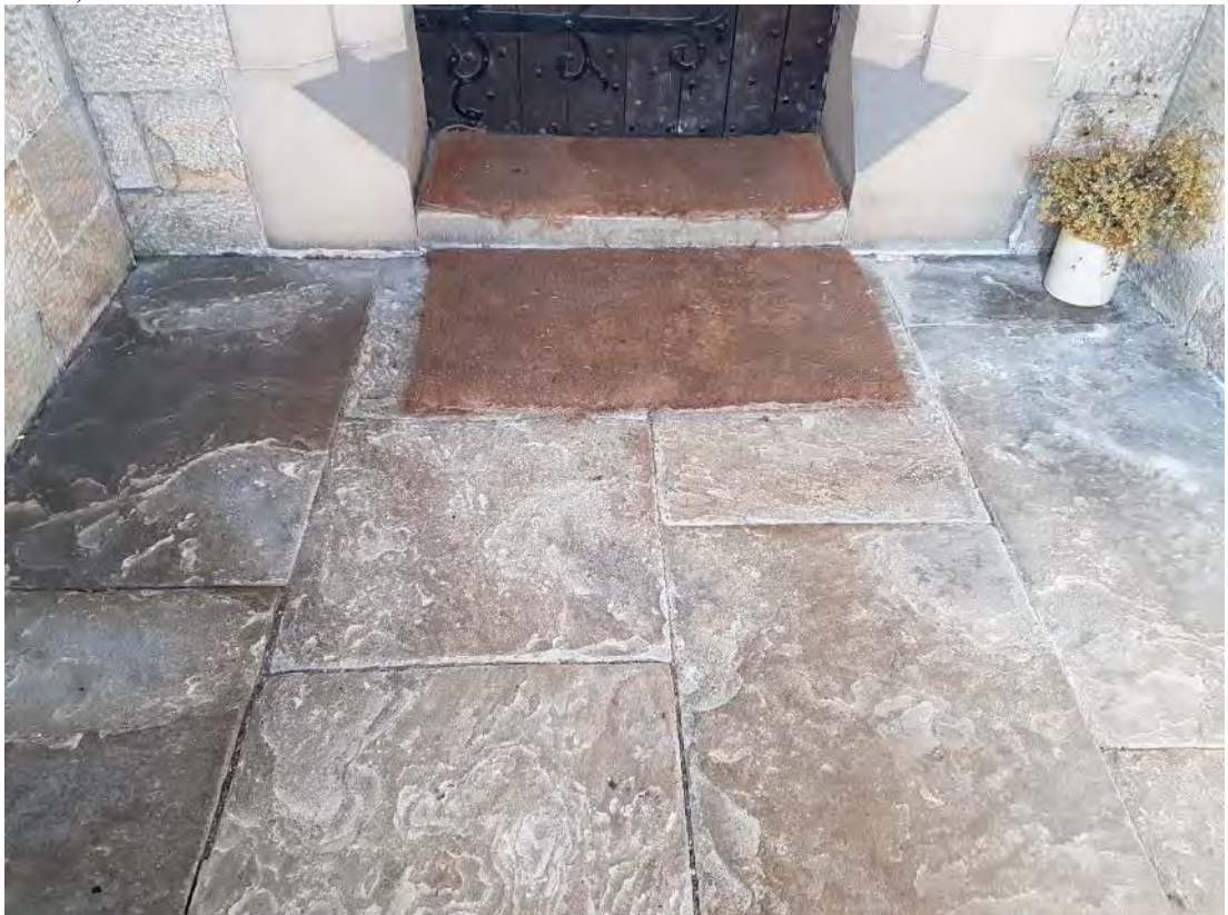
Figure 72: The limestone slabs of the flooring of the porch (Source: Author 2019).
