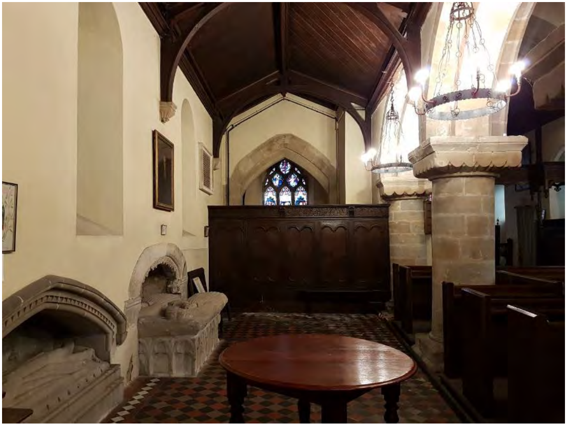
Figure 79: The north aisle, looking east, showing the top of the double-chamfered pointed arch between the chancel bay/vestry and eastern nave bay of the north aisle, as well as the altered and reused seventeenth-century screen (Source: Author 2019).
