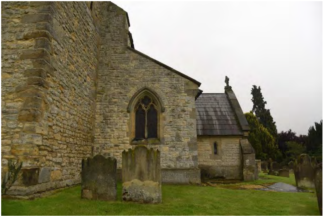
Figure 50: The western elevation of the southern aisle, showing a Victorian Middle Decorated Gothic pointed window, comprising a two-light window with trefoil heads and a central quatrefoil above. The window has an alternating straight and hollow-chamfered surround comprised of stone quoining, with a chamfered sandstone sill. The rounded hood-moulds terminate in moulded label stops (Source: Author 2019).
