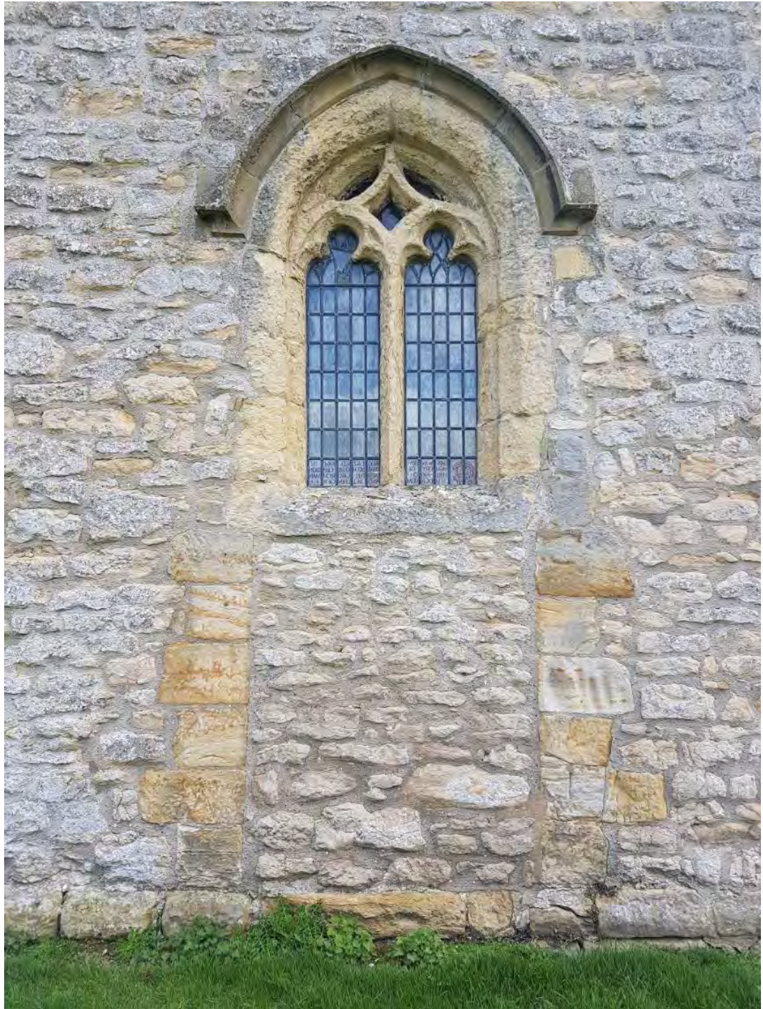
Figure 114: first stage of the western elevation has a twelfth-century quoin doorway filled with rubble masonry with a fifteenth-century Decorated Gothic pointed arch window above. The infill of the doorway is likely to be contemporary with the window (Source: Author 2019).
