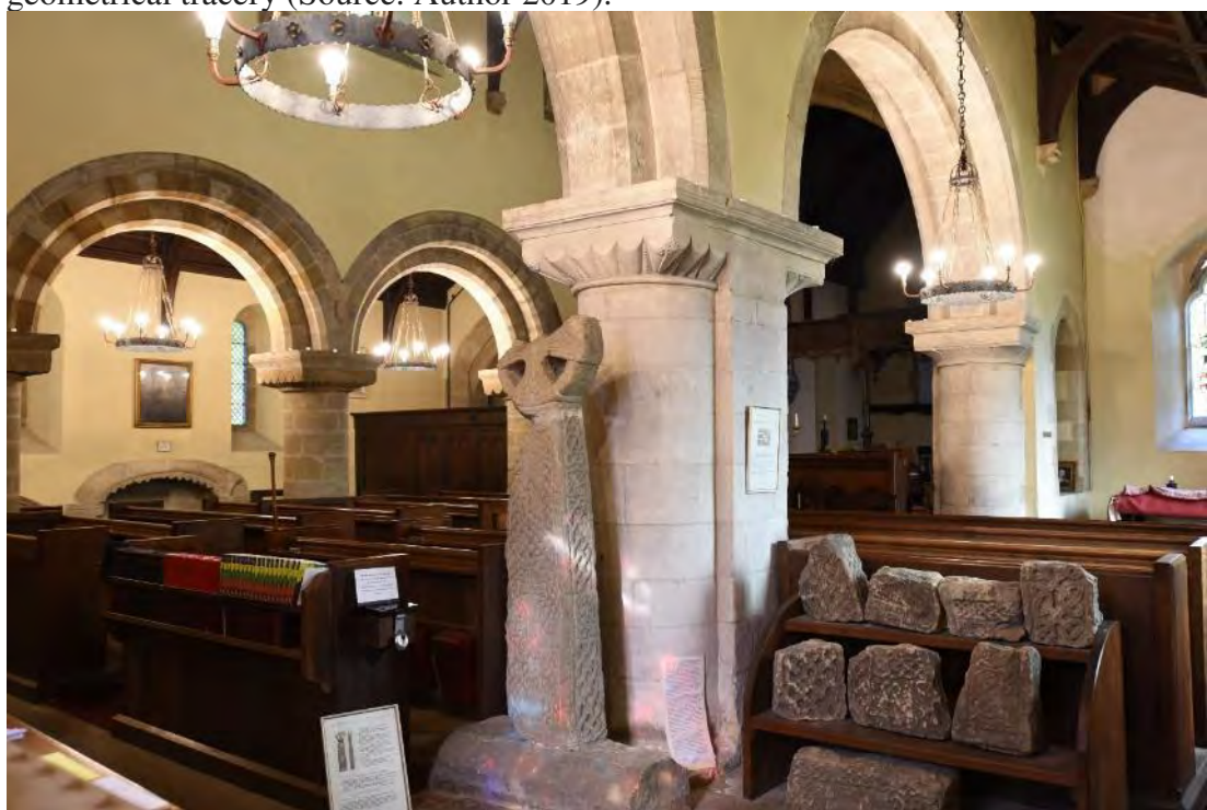
Figure 53: The three bays of the northern side of the south aisle, showing the two arcades and the opening in the eastern chapel, with the north aisle in the background (Source: Author 2019).
