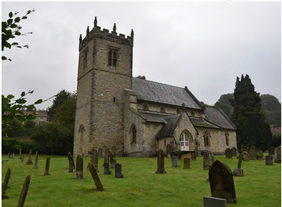
Figure 139: Photograph from 2019 showing the exterior of the church from the south-west, showing the retained tower but rebuilt aisles, chancel and roofing. The photograph has been taken north of the stone walls due to foliage growth obscuring the view from the location of the 1862-3 photograph (Source: Author 2019).
