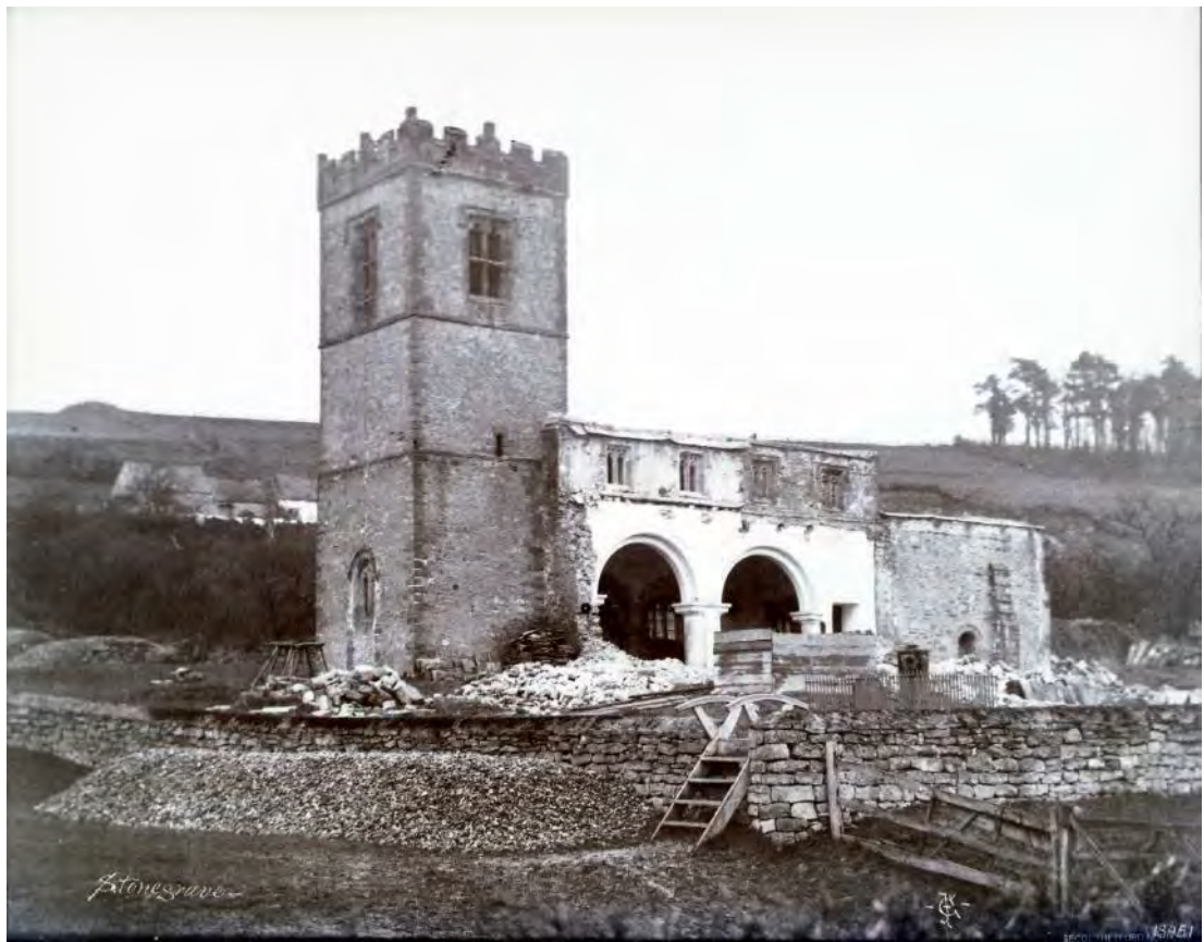
Figure 138: Photograph by G.F. Jones during the 1862-3 restoration, showing the exterior from the south-west; note the C12 arcades, square-headed door, C15 clerestory, C11/C12 chancel and whitewashed interior Source: NSM RPS 18951).
