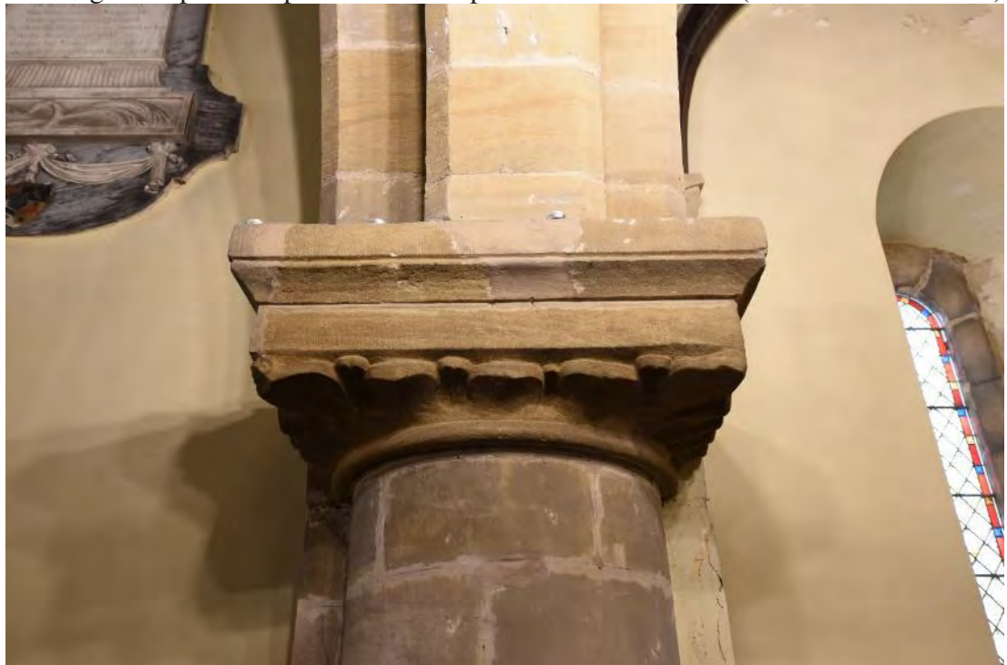
Figure 24: The capital of the western pillar of the western bay of the north arcade, between the western nave wall and the northern aisle, showing the use of two orders in the one capital: scalloped trumpets on the northern and eastern edges; and, a waterleaf capital on the eastern edge (Source: Author 2019).
