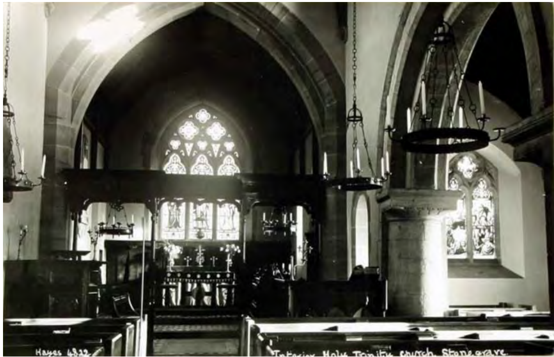
Figure 63: 1945 photograph of the nave, chancel and eastern end of the south aisle, showing the east-facing pews in the south aisle prior to the 1960s conversion into a chapel, as well as the Victorian chandeliers with candles, prior to their retrofitting and relocation (Source: HEA 6433_066).
