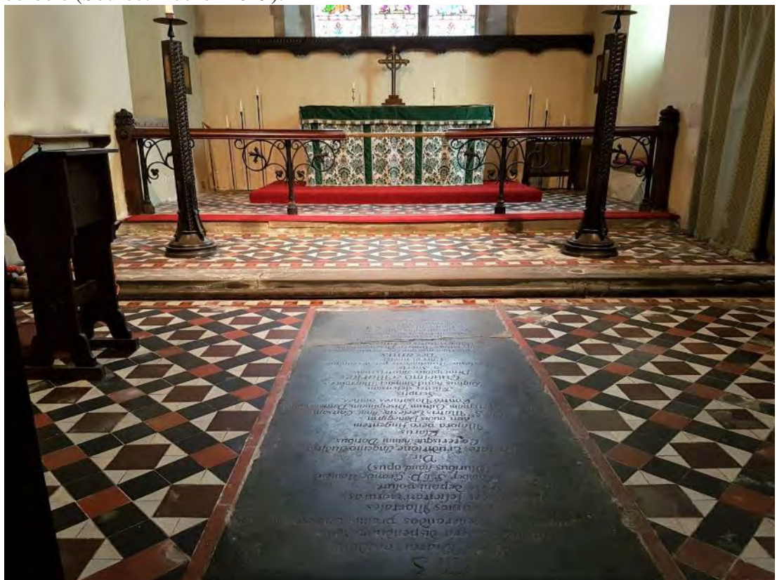
Figure 107: The floor of the chancel is composed of three equally spaced steps rising up to the altar, with bare limestone slabs at each step but with the rest of the floor covered with geometric tiles, with Dean Thomas Comber's gravestone in the western bay (Source: Author 2019).
