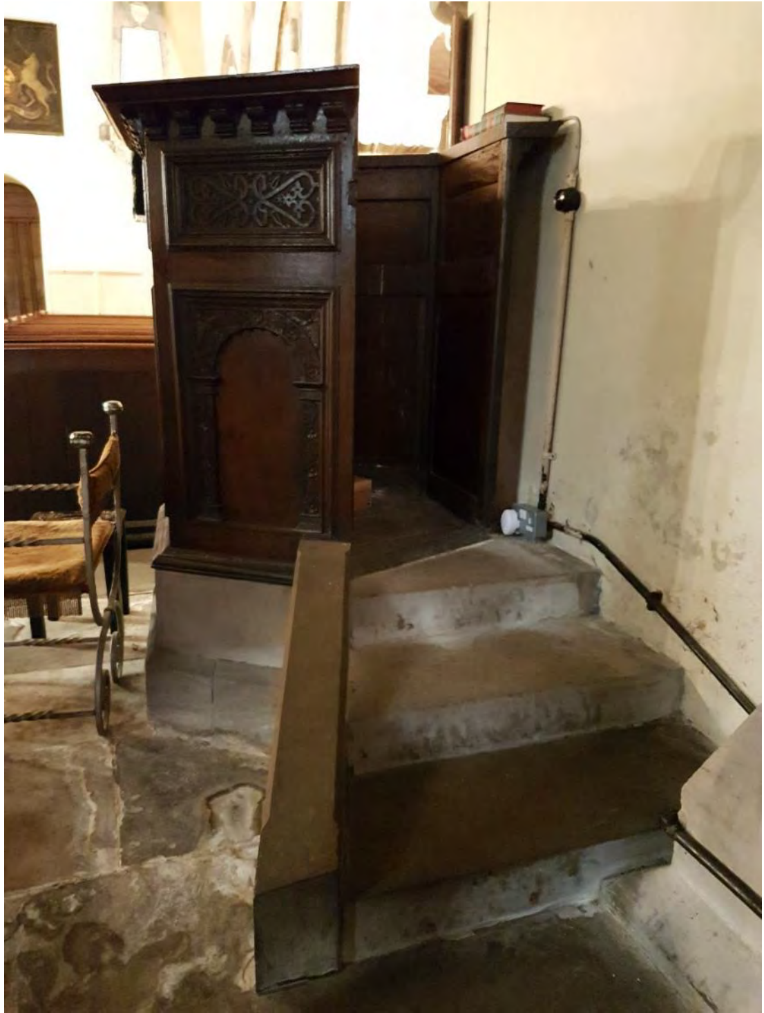
Figure 46: The pulpit at the north-eastern corner of the nave, showing the seventeenth-century pulpit to have been reused, set onto a 1862-3 sandstone base, taken from the east (Source: Author 2019).
