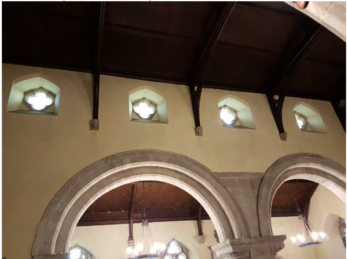
Figure 41: The C15 corbels along the south clerestory wall clerestory windows, displaying human heads, interspersed between windows of quatrefoil tracery set inside a chamfered segmental pointed arched surround and chamfered sill (Source: Author 2019).
