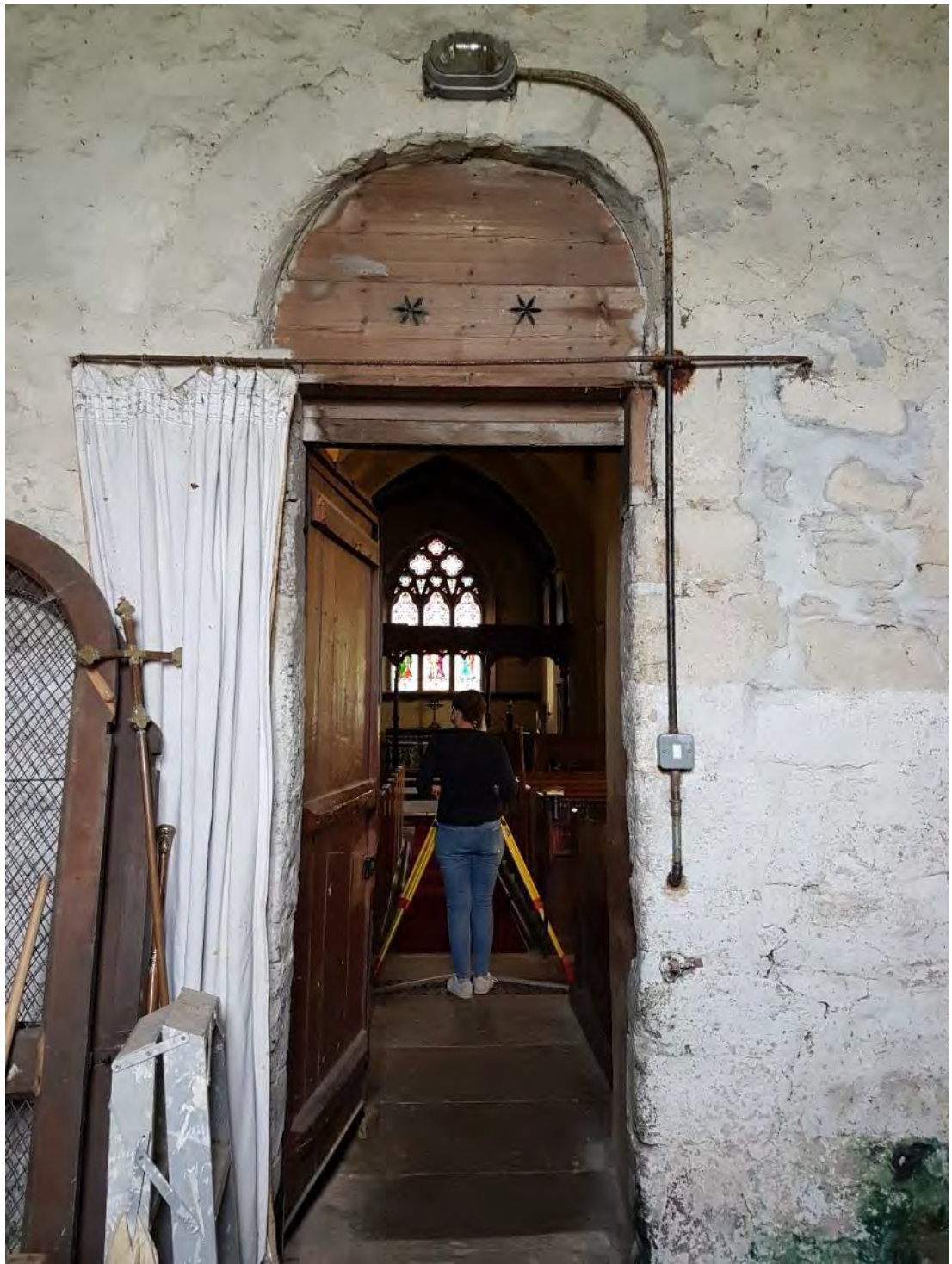
Figure 37: The western side of the Saxo-Norman door from inside the tower, looking east (Source: Author 2019).
