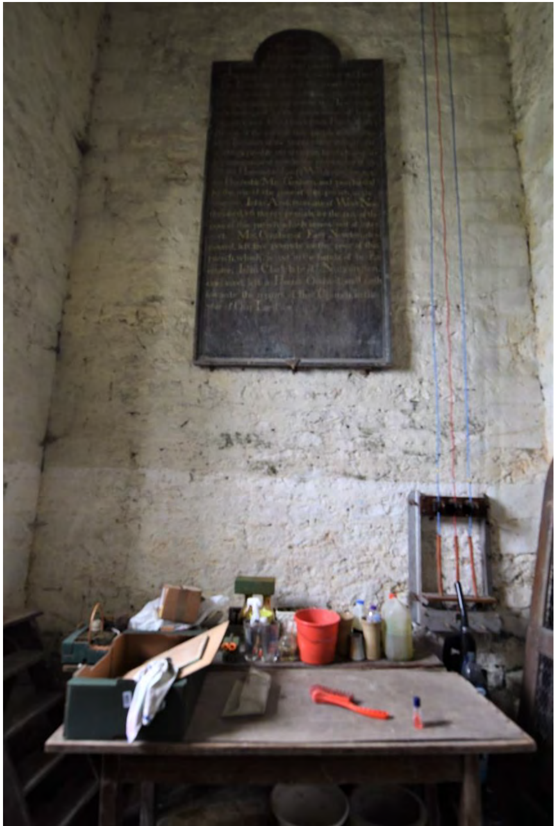
Figure 117: The northern interior wall of the first stage of the western tower, showing the eighteenth-century benefactors' board fixed to the wall, as well as the painted coursed rubble masonry (Source: Author 2019).
