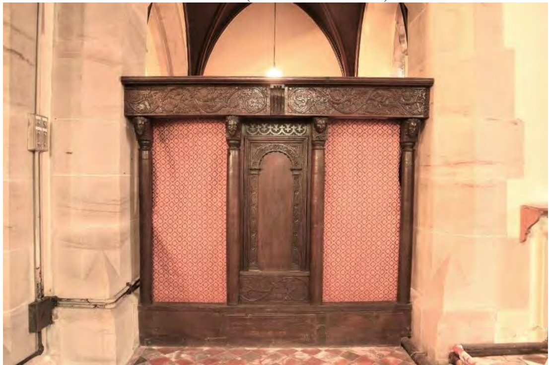
Figure 184: The seventeenth-century screen/panelling separating the chancel bay and chancel, comprising the floriated frieze along the top, column shafts topped with heads, a central panel with a decorative arch and plain panelling at the base (Source: Author 2019).
