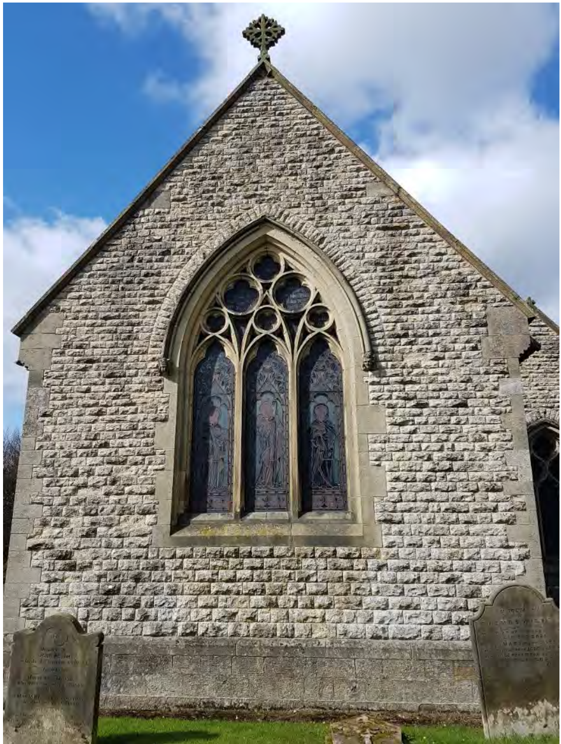
Figure 92: The eastern elevation of the chancel, showing the three-light Victorian Middle Decorated Geometric Gothic pointed arch window with cusped heads and quatrefoil and trefoil tracery and rounded hood-moulds with head-stops, as well as a sandstone coping with a decorative cross finial and moulded kneelers (Source: Author 2019).
