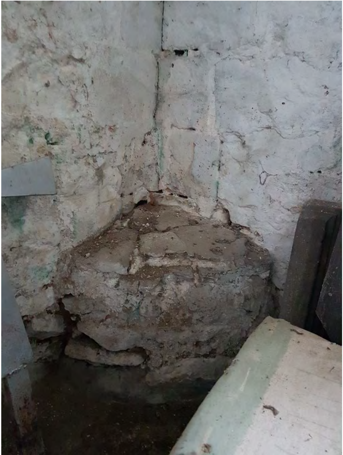
Figure 124: The south-west tower platform (Source: Author 2019).
