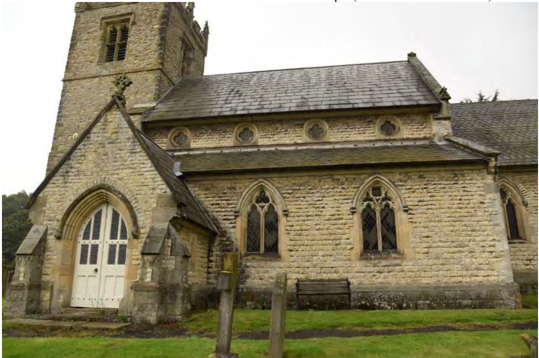
Figure 51: The southern elevation of the southern aisle, showing a porch in the western bay and Victorian Middle Decorated Gothic pointed windows in the eastern two bays. Both windows comprise two-light windows with trefoil heads and alternating trefoil and quatrefoil geometrical tracery (Source: Author 2019).
