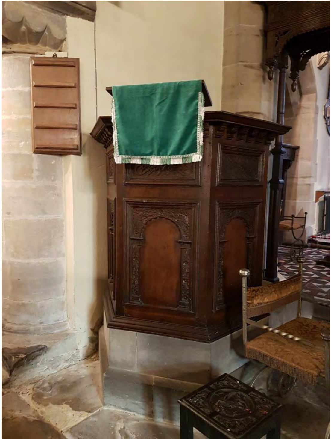
Figure 45: The pulpit at the north-eastern corner of the nave, showing the seventeenth-century pulpit to have been reused, set onto a 1862-3 sandstone base, taken from the south-west (Source: Author 2019).
