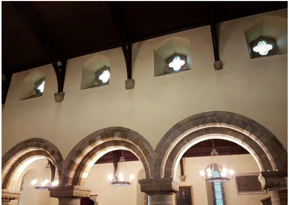
Figure 162: The reused C15 corbels along the north wall of the 1862-3 clerestory, decorated with family crests and human heads. The corbels have been reused at a lower height than for the C15 clerestory (Source: Author 2019).
