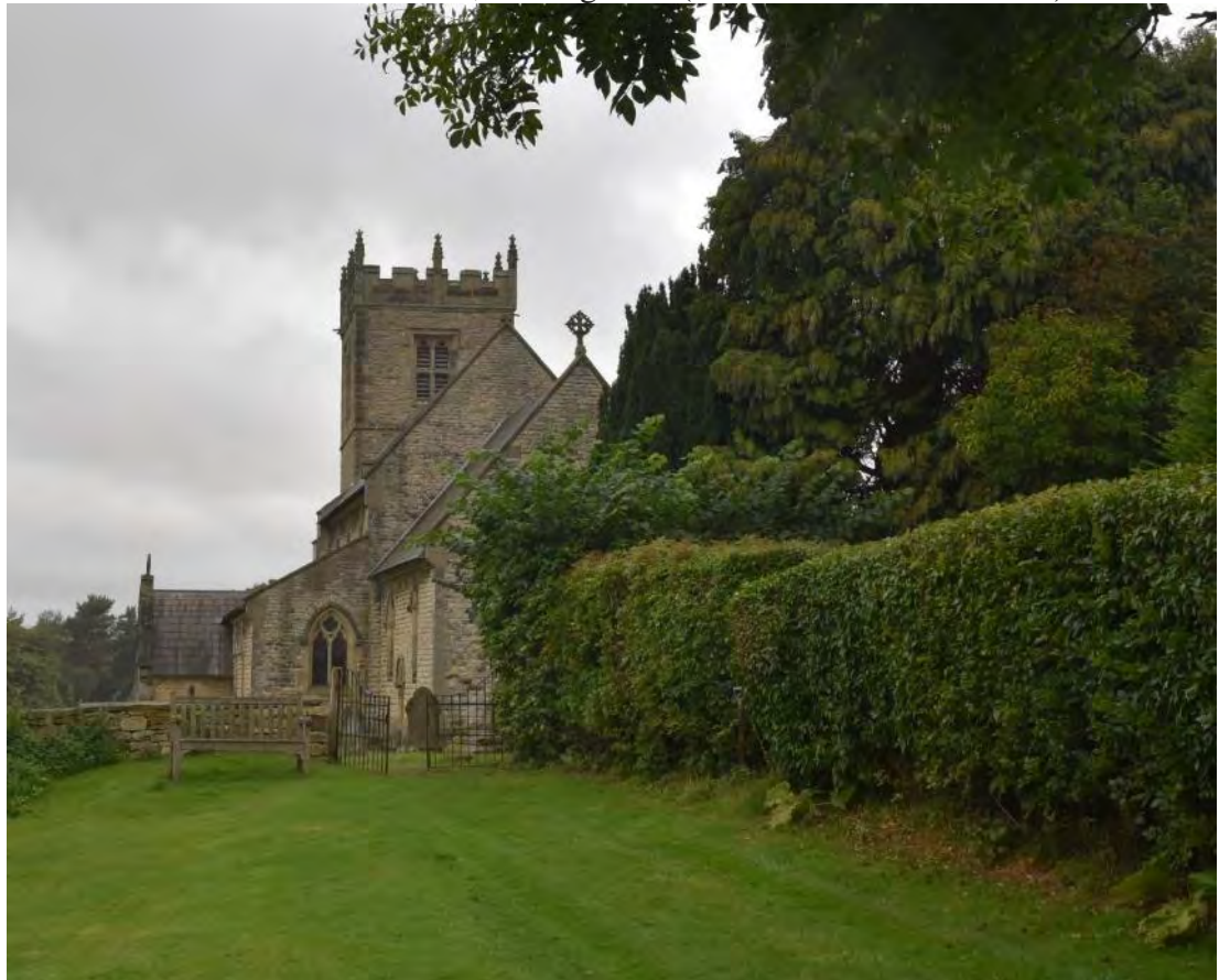
Figure 137: Photograph of the eastern elevation in 2019, looking west (Source: Author 2019).
