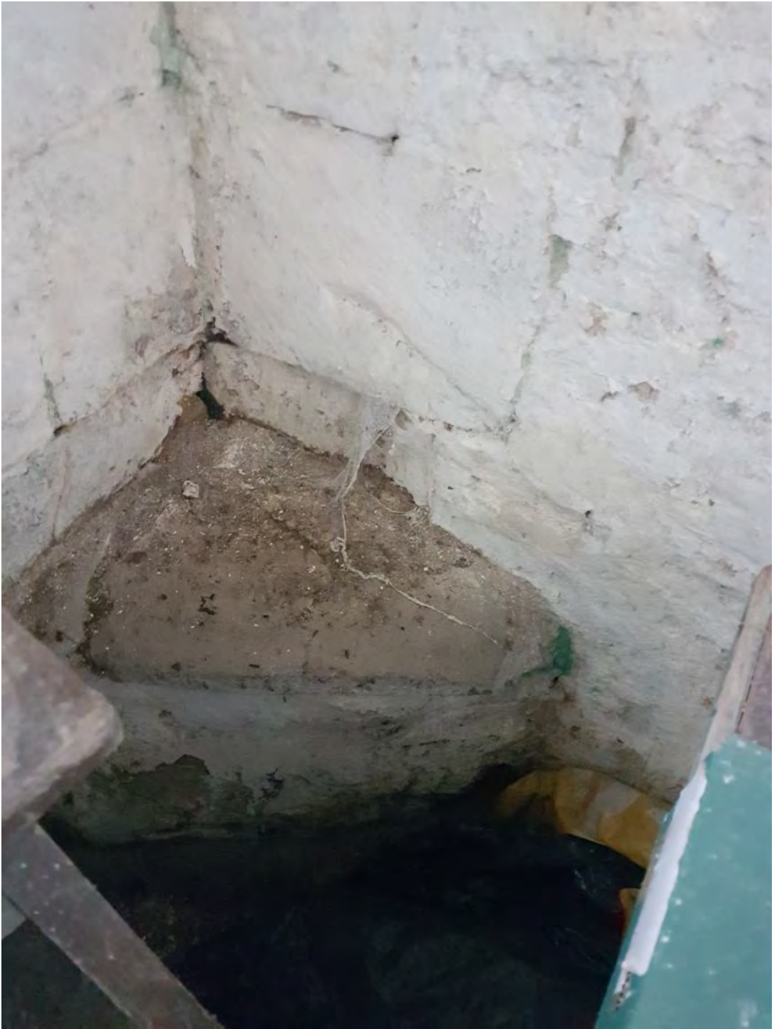
Figure 123: The north-west platform in the tower (Source: Author 2019).
