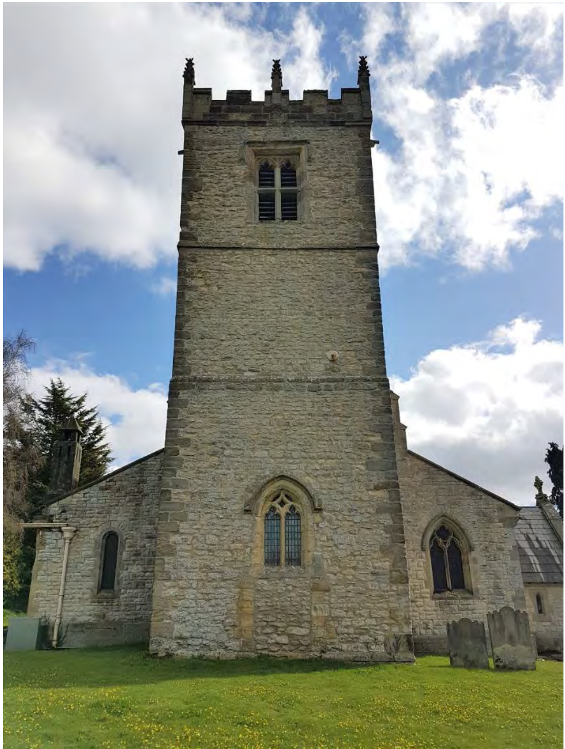
Figure 110: The western elevation of the three-stage square tower, constructed from coursed rough limestone rubble with dressed calcareous sandstone quoining, showing the location of the fifteenth-century Perpendicular window blocking the head of the earlier twelfth-century door (Source: Author 2019).
