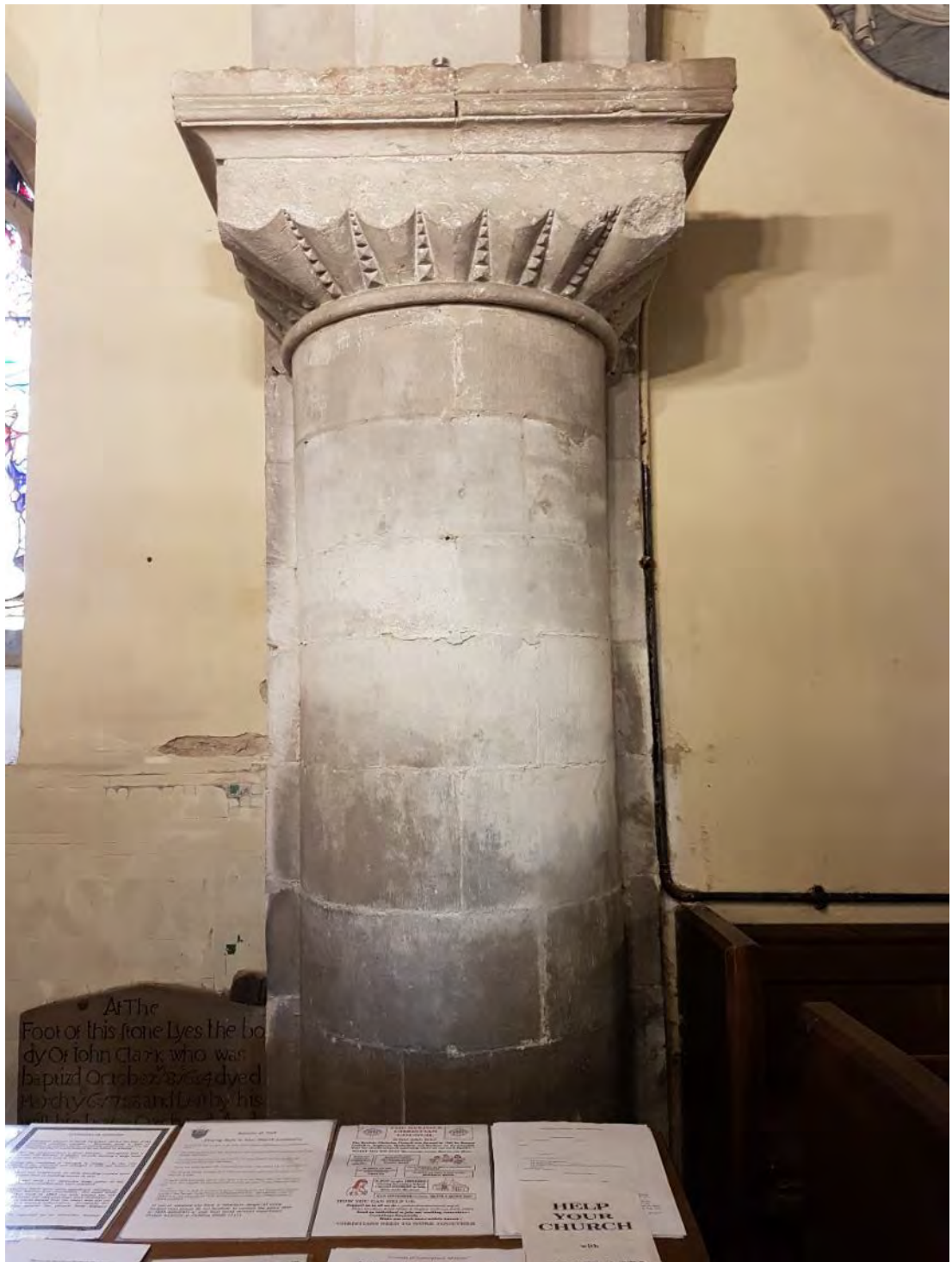
Figure 29: The western column of the western bay of the arcade, showing the scalloped trumpet capital with nailhead decoration between the scallops (Source: Author 2019).
