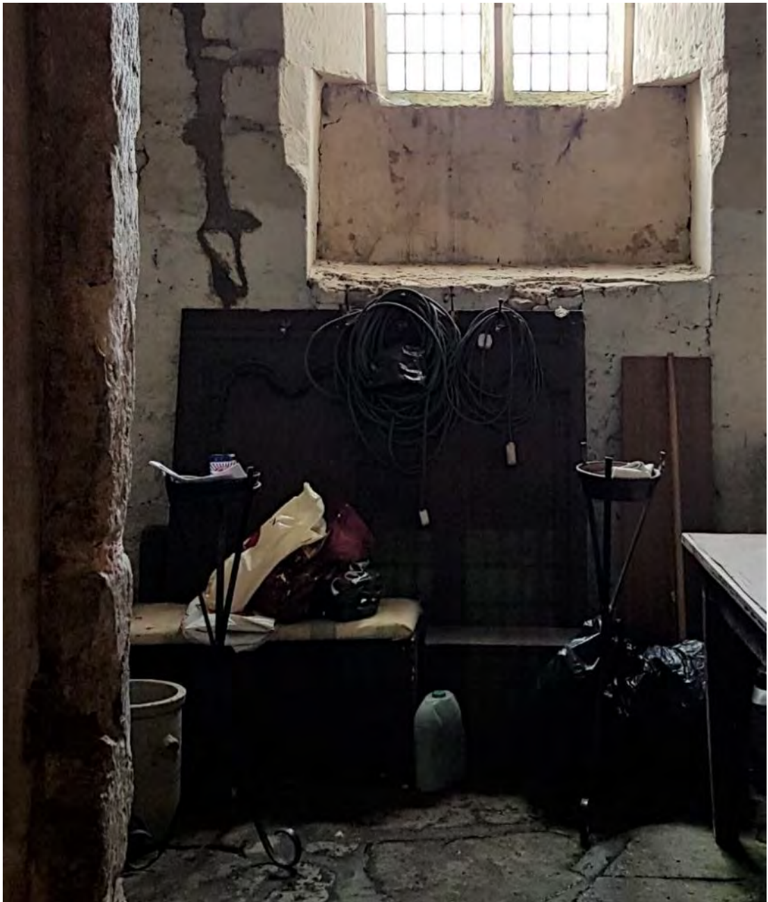
Figure 186: A currently unmounted section of seventeenth-century panelling along the western wall of the tower, showing the double-arched panels, with later fixings along the top for hanging items (Source: Author 2019).
