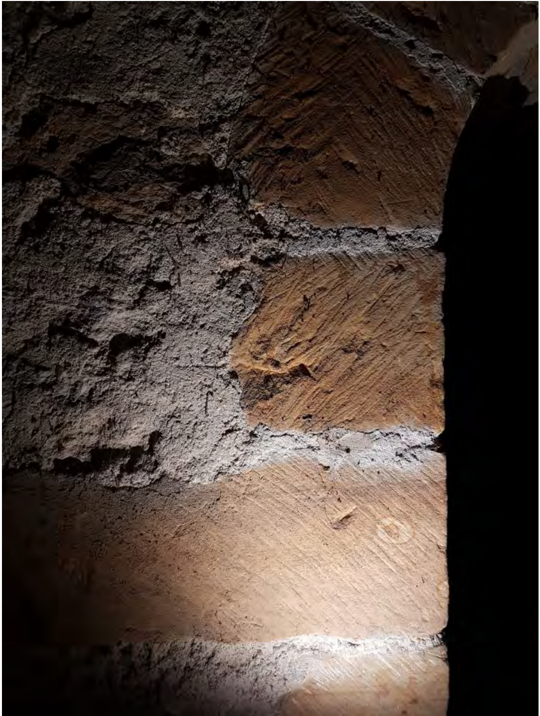
Figure 133: The twelfth-century oblique tooling in the surround for the Norman door in the eastern wall of the second stage of the tower (Source: Author 2019).
