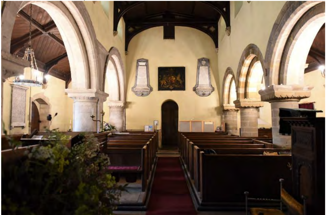
Figure 13: The interior of Stonegrave Minster, taken from the entrance to the chancel and showing the retained medieval fabric of the arcades in the nave and the entrance to the tower (Source: Author 2019).
