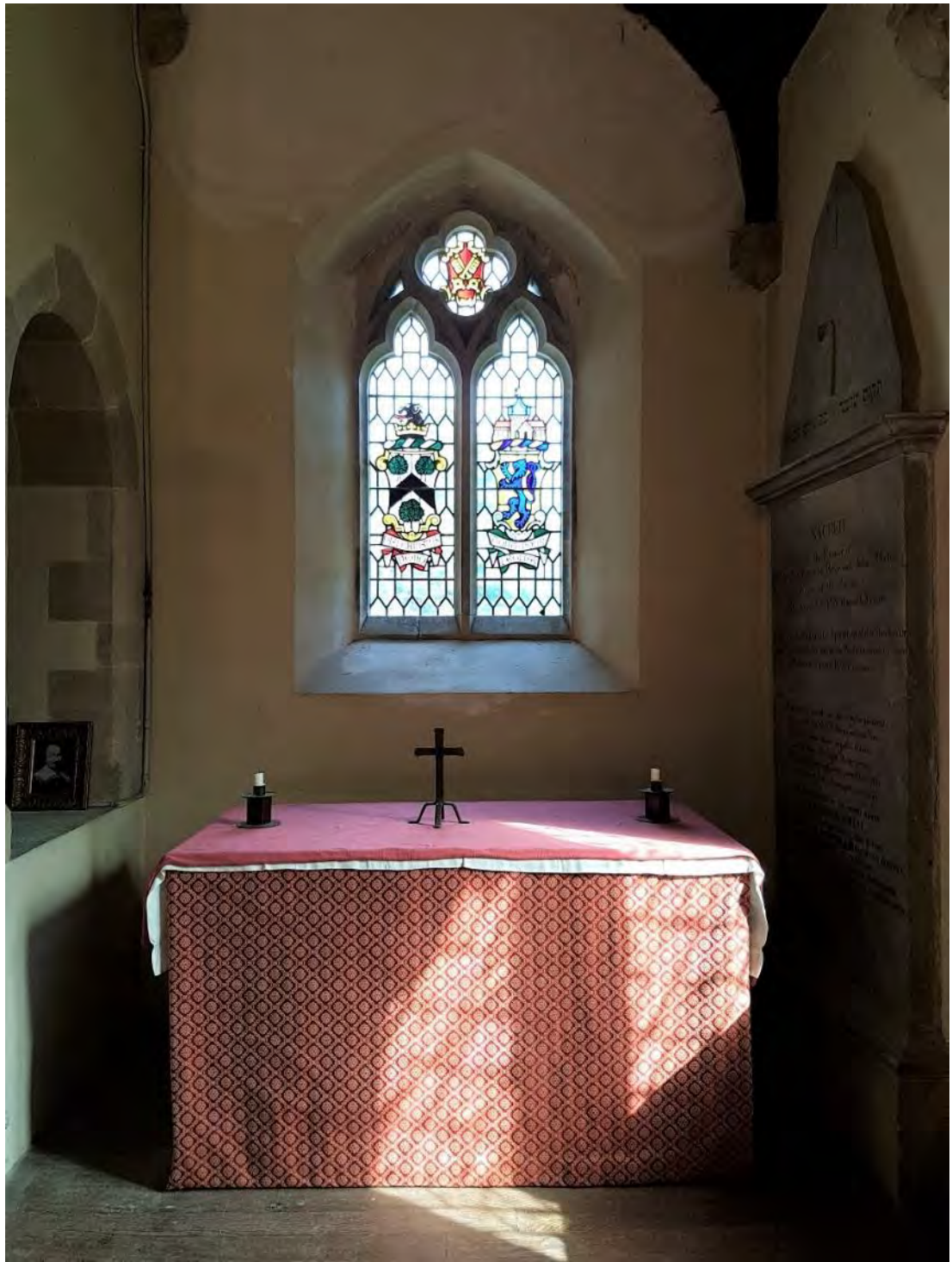
Figure 61: The chapel in the eastern bay of the south aisle, showing from the left: the squint in the north wall between the nave and the chapel; the Victorian Middle Decorated Gothic pointed arch window of the western elevation; the reused C17 altar below; and, the C19 memorial on the southern wall (Source: Author 2019).
