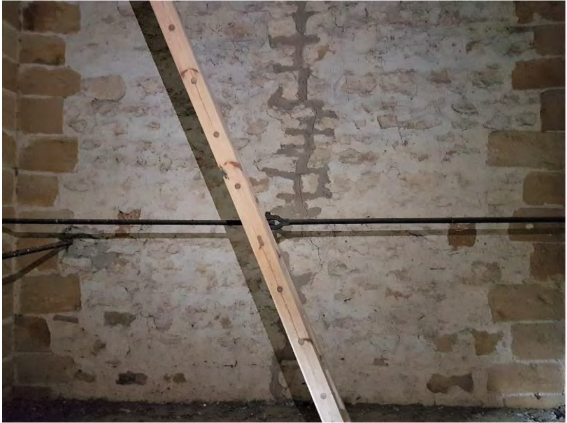
Figure 129: The plastered coursed rubble stone masonry with exposed sandstone quoining in the second stage of the tower (Source: Author 2019).
