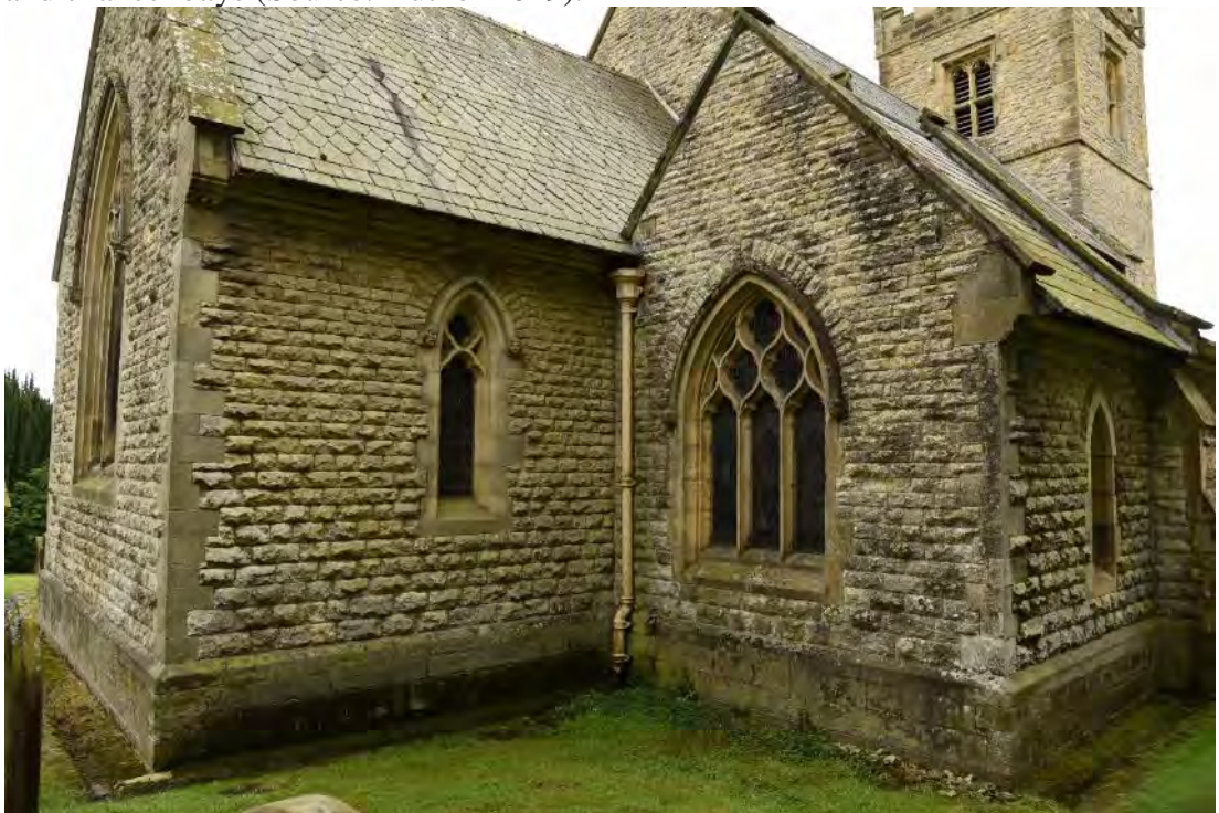
Figure 76: The eastern elevation of the north aisle, showing the three-light Victorian Decorated Geometric window, next to the northern elevation of the chancel (Source: Author 2019).
