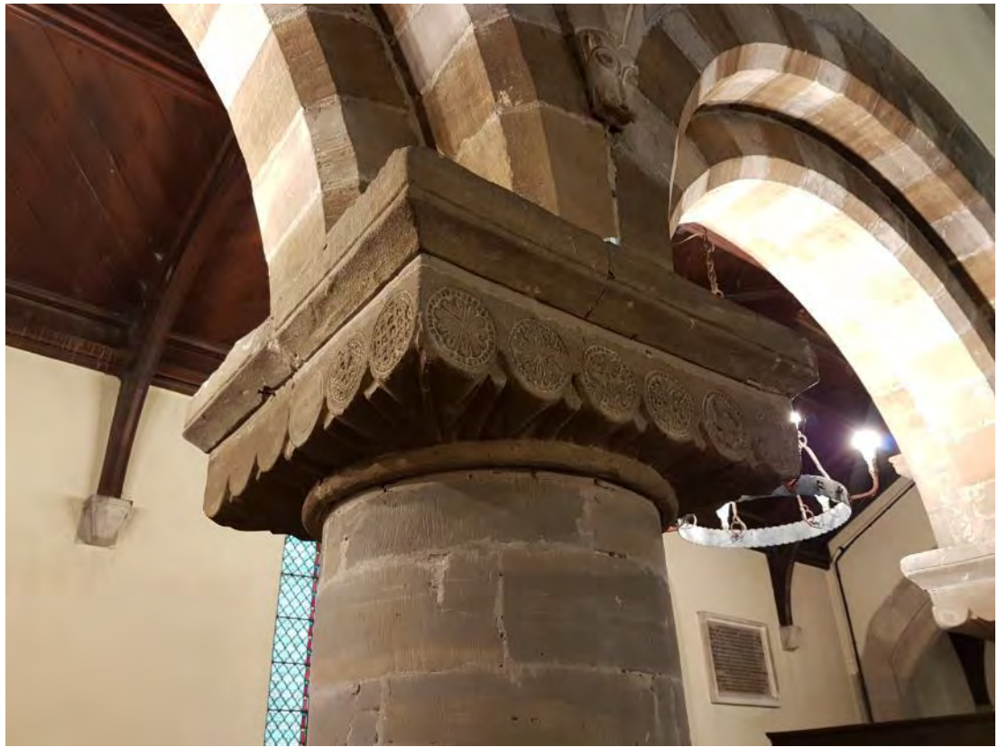
Figure 23: The capital of the western pillar of the central bay of the northern arcade, showing scalloped trumpets with incomplete floral medallions (Source: Author 2019).
