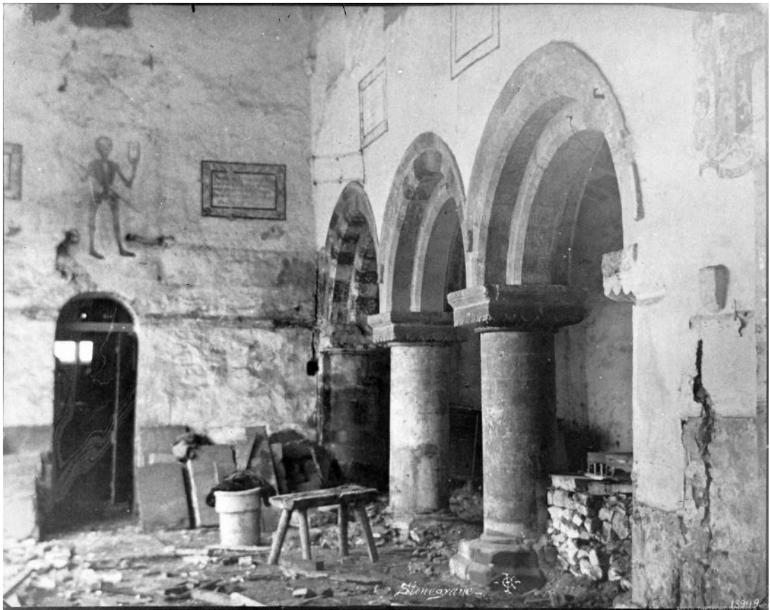
Figure 144: Photograph taken during the 1862-3 restoration, showing the interior, demonstrating the scriptural texts, the coat of arms above the pulpit, the 'time and death' painting and shadows of a western gallery (Source: NSM RPS 18949).
