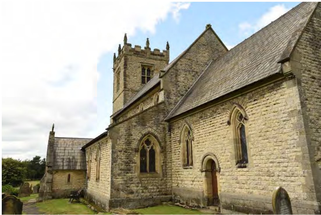
Figure 52: The eastern elevation of the southern aisle, showing a two-light Victorian Middle Decorated Gothic pointed arch window with trefoil heads and quatrefoil geometrical tracery (Source: Author 2019).
