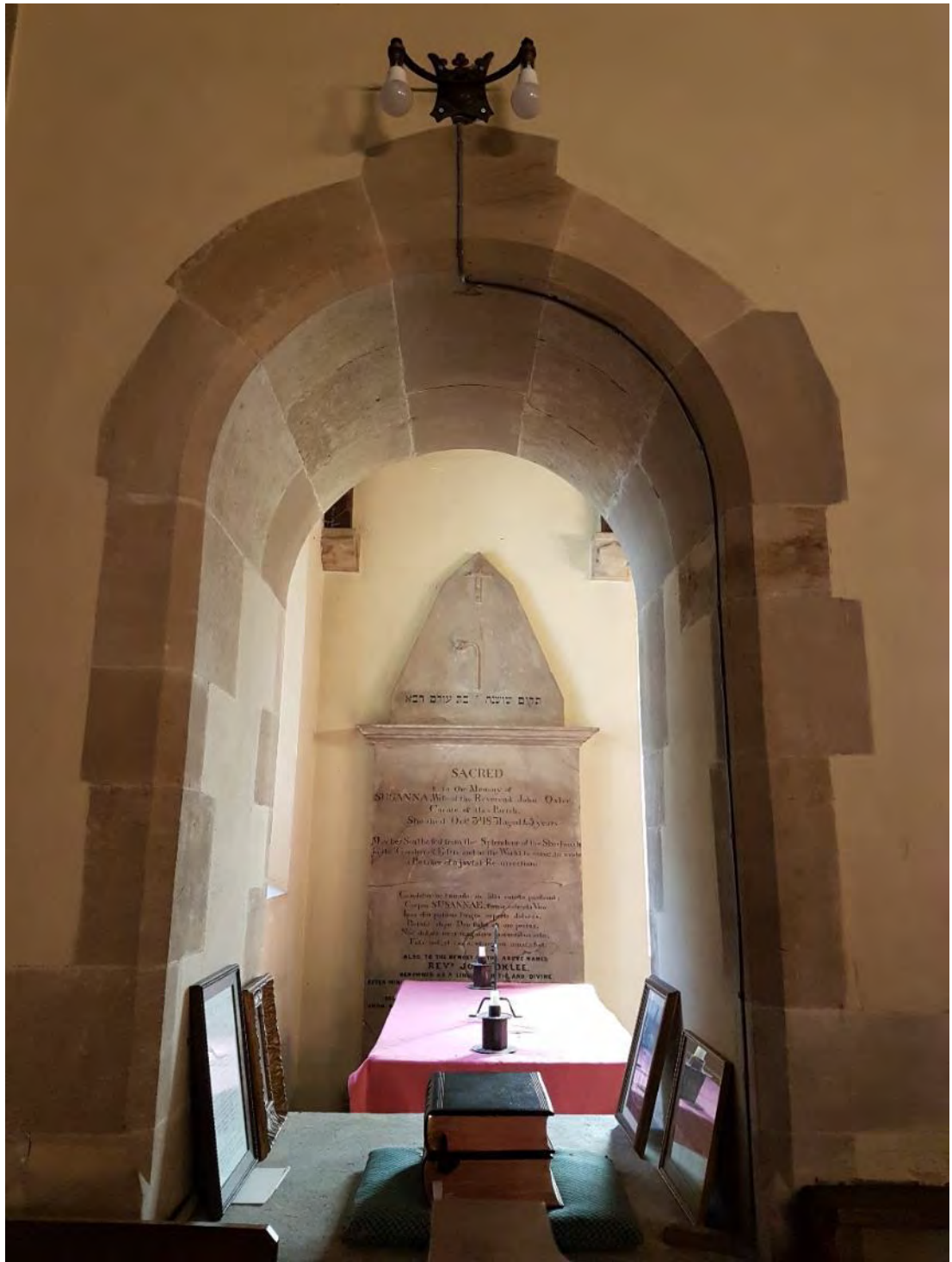
Figure 28: The eastern opening the southern wall of the nave, looking through to the altar in the south aisle, comprising a chamfered round-headed window using smooth-faced stone quoining and a solid stone block sill (Source: Author 2019).
