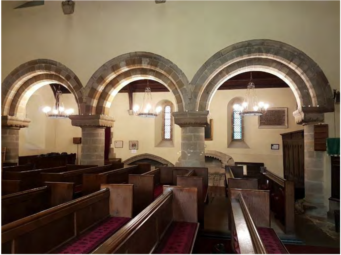
Figure 77: The view of the interior of the north aisle from the nave, showing the Norman arcade along the south of the aisle and the two lancet windows in the northern elevation (Source: Author 2019).
