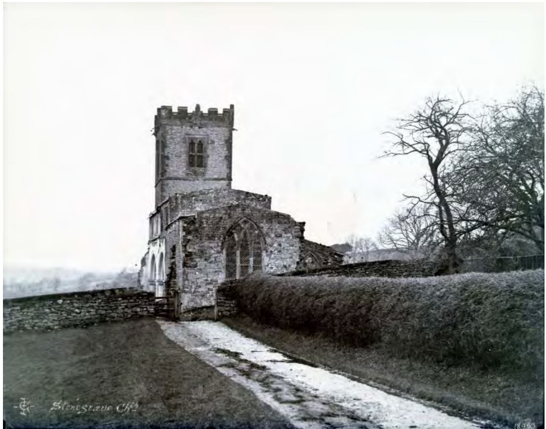
Figure 14: Photograph by George Fowler Jones during the 1862-3 restoration, showing the C15 roof structure of the chancel and nave, looking west. It also shows that the southern aisle was fully demolished (Source: NSM RPS 18950).
