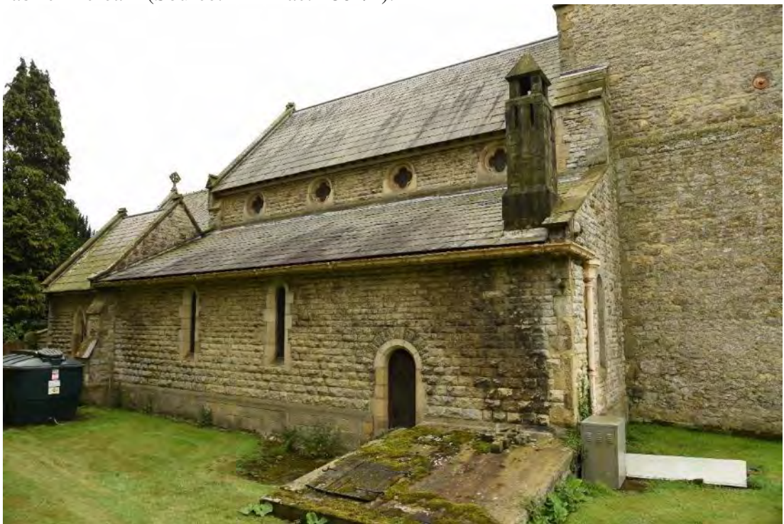
Figure 166: The existing northern aisle, showing the Norman door in the western bay and lancet windows in the central and eastern bays of the nave aisle, with the chancel bays at the far left (Source: Author 2019).
