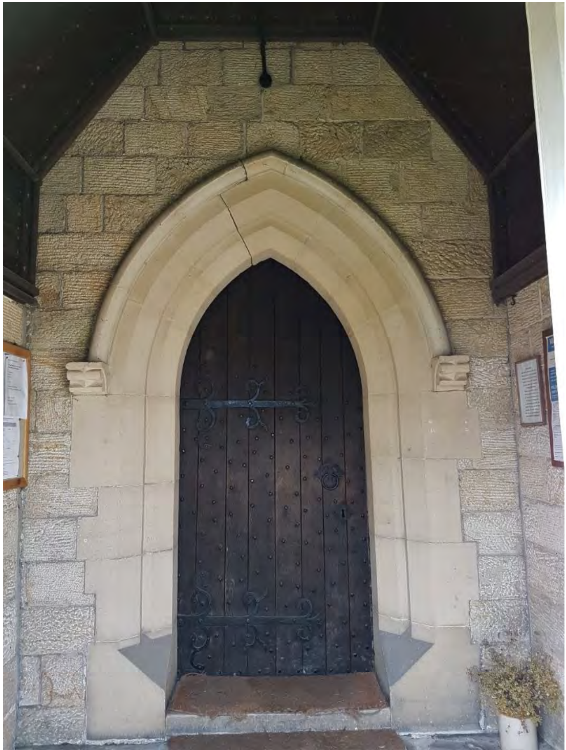
Figure 68: The northern internal elevation of the porch, showing the double-chamfered pointed arch door between the porch and south aisle, as well as the stone courses from the west and east walls not matching up with those of the north wall (Source: Author 2019).
