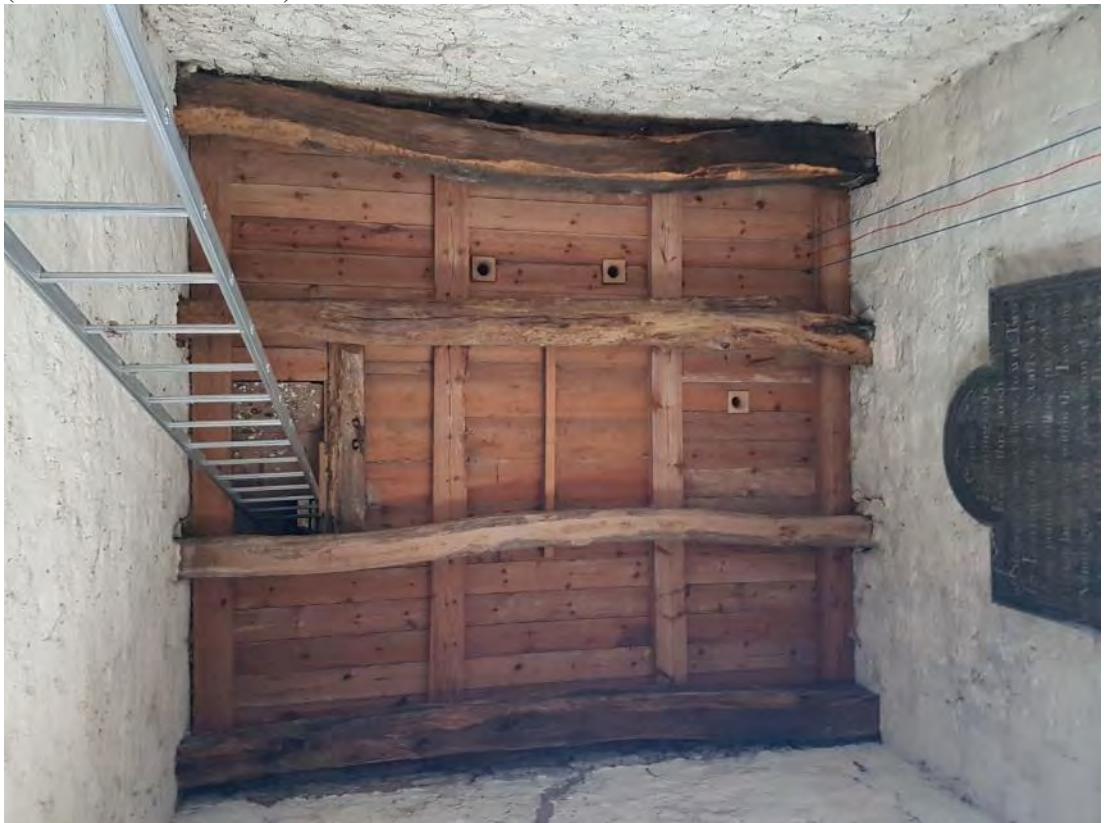
Figure 128: The 1885 timber platform for the second stage of the tower, taken from below in the first stage (Source: Author 2019).
