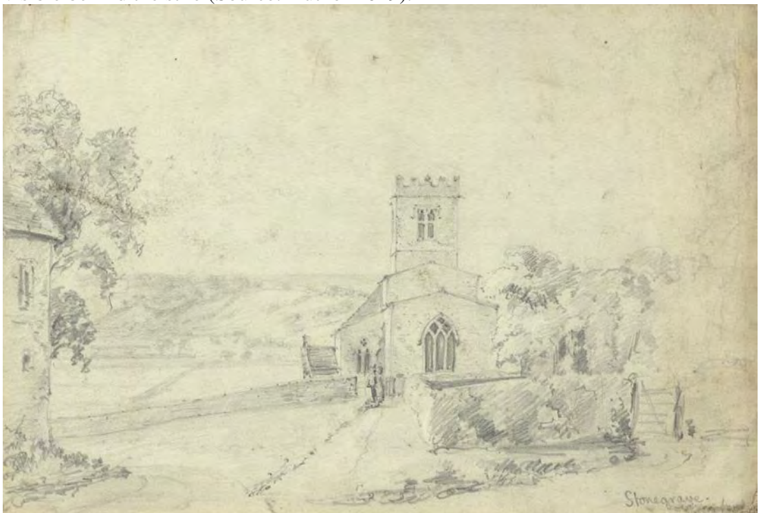
Figure 141: Nineteenth century graphite sketch, looking west towards the eastern elevation of the church, showing the pre-restoration chancel, south aisle and porch, as well as the C15 low pitched roofing, the C13 Decorated Geometric window of the south aisle, the C18 intersecting y-tracery of the eastern window and the curious steep-pitched roof of the western section of the south aisle (Source: Somerset and Wood 2016).
