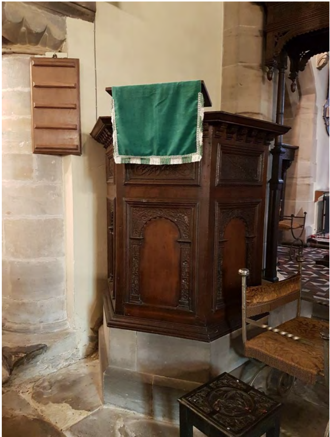
Figure 153: The extant pulpit at the north-eastern corner of the nave, showing the 1637 pulpit to reused and set onto an 1862-3 sandstone base (Source: Author 2019).
